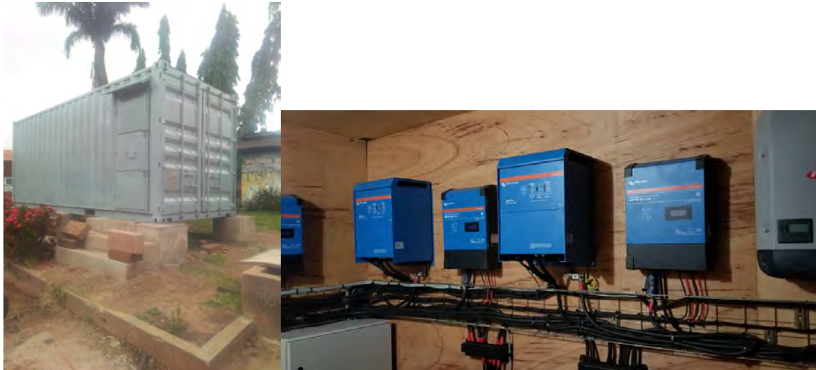
Figure 1: Indoor & Outdoor of container 1
