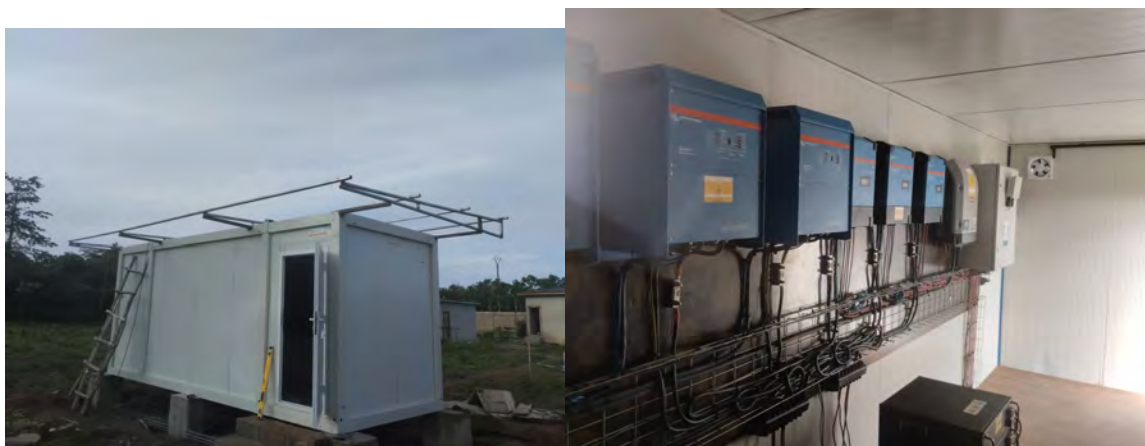
Figure 2: Indoor & Outdoor of container 2
