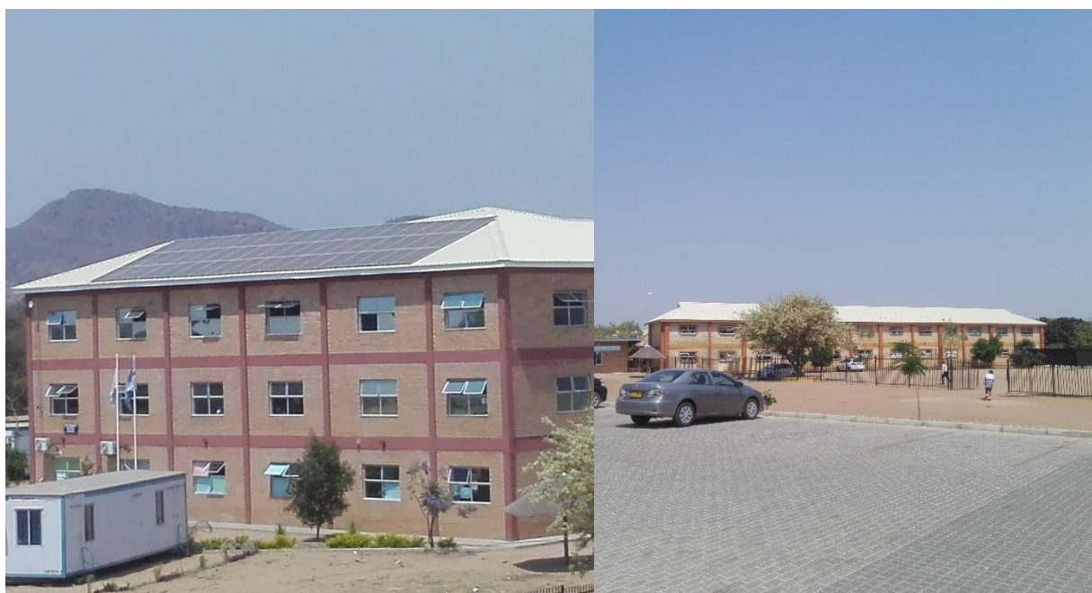
Figure 7. Regent Hill School Energy Village
