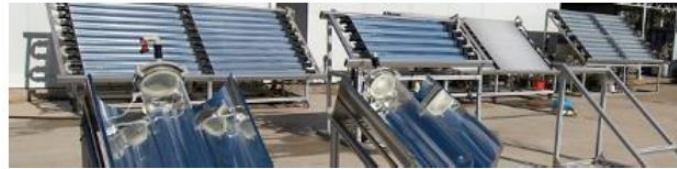
Figure 8: Water purification solar prototypes (reactors) located at CIEMAT-PSA
